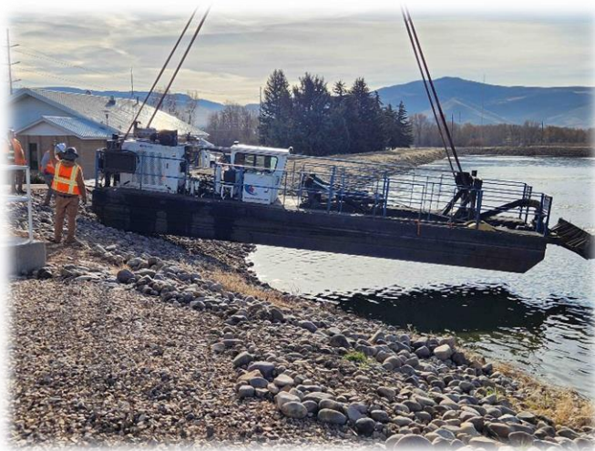
Dredge being placed in Lagoon Cell 1
