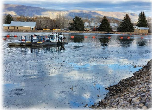
Dredge with Floating Slurry Pipe (Note Solids Processing Area in Background)
