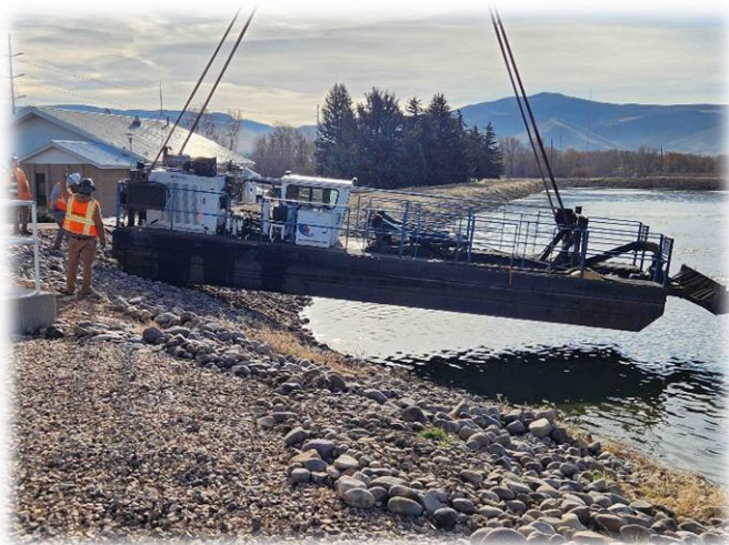
Dredge being placed in Lagoon Cell 1
