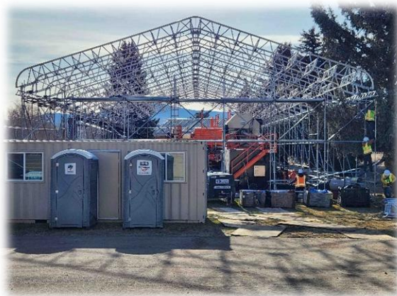
Tent Structure Being Erected Over Solids Processing Area
