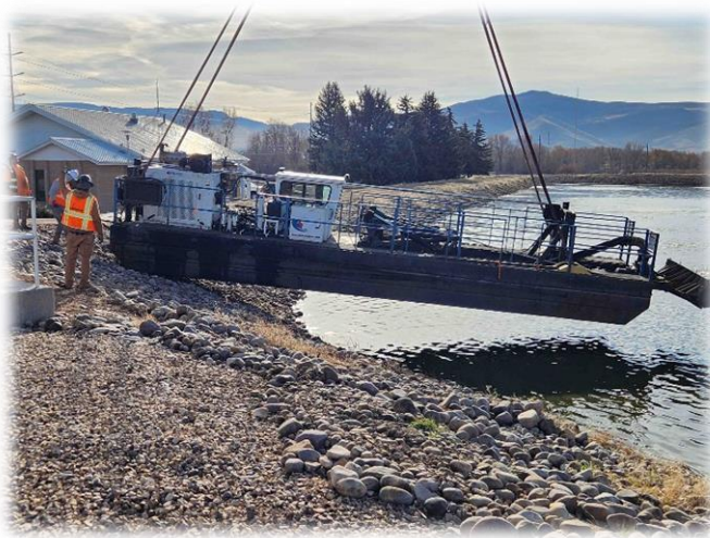
Dredge being placed in Lagoon Cell 1
